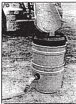
Figure 3. Concrete washout filter
