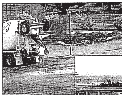
Figure 1. Chute washwater being dumped on the ground
